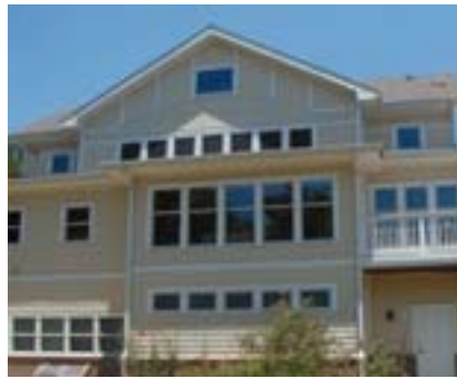
The south side of the Southface office building uses passive solar design. In the winter, the sun shines on the windows and warms the living space, reducing the heating load on the building. In the summer, overhangs shade the windows, reducing the cooling load on the building.
