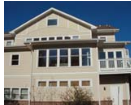
The south side of the Southface office building uses passive solar design. In the winter, the sun shines on the windows and warms the living space, reducing the heating load on the building. In the summer, overhangs shade the windows, reducing the cooling load on the building.
